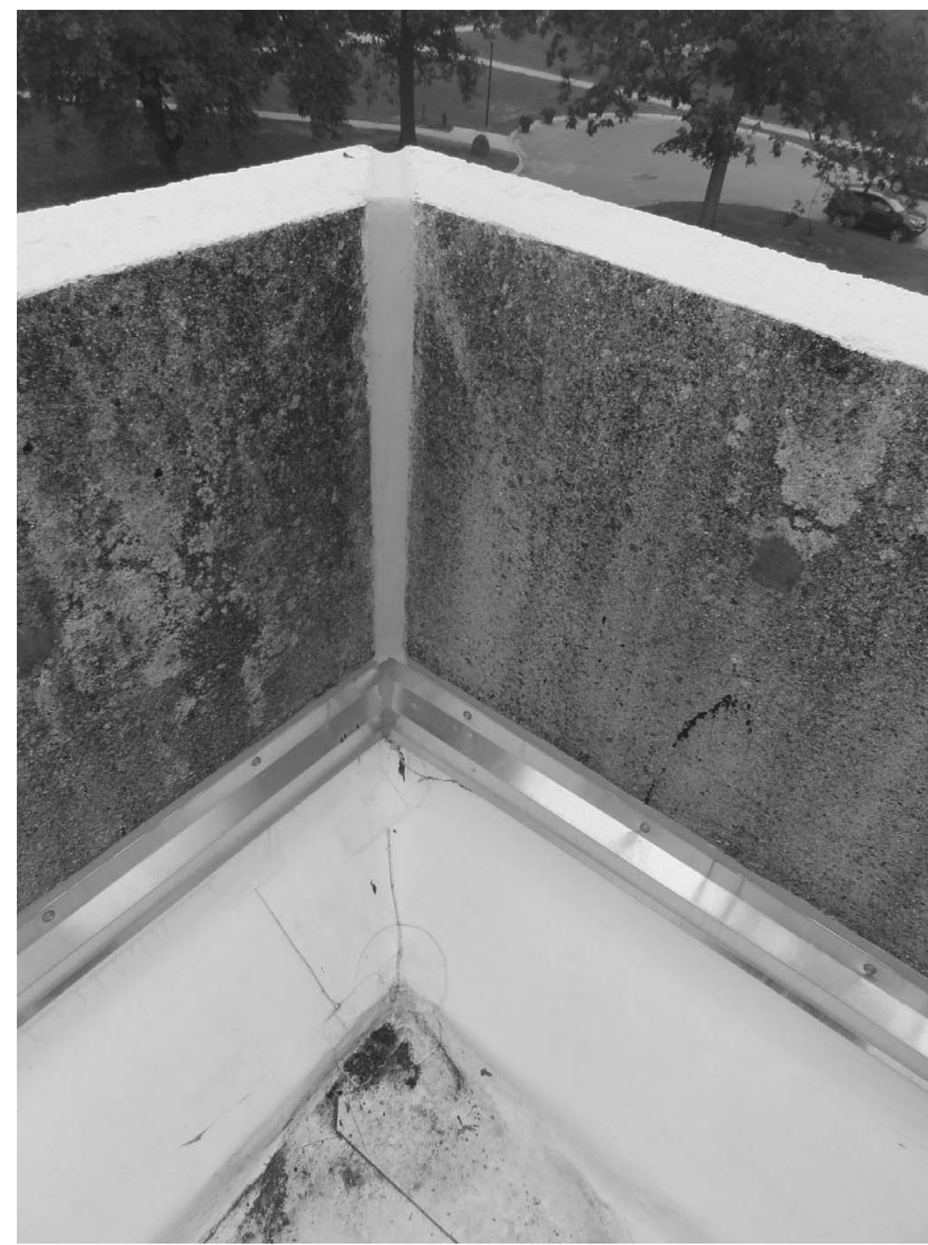
STANLEY HALL PARAPET EXISTING CONDITIONS PHOTO PANEL JOINT AT OUTSIDE CORNER
